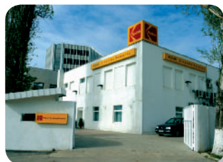
Below: Cinelabs Romania
